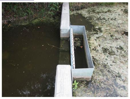
Fish grate partially blocking flow, water 3" above weir, with stains 3" higher
