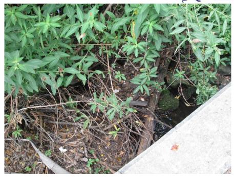
Trapped debris in front of headwall on Wingspan Way, east of Covey Ct
